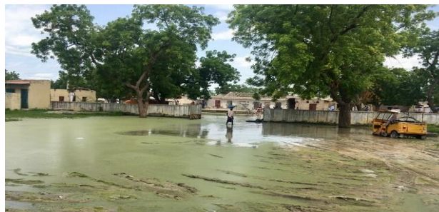
A PHC facility surrounded by stagnant water during rainy season which can become a mosquito breeding ground.
